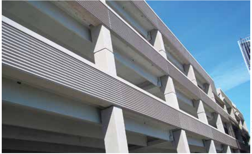
The terra cotta panels used on the Logan CONRAC project provided warmth and texture in a panelized system that was easy to erect. The sheets were 3/4-inches thick and measured 2 by 3 feet. Using embedded terra cotta saved about $1 million, according to the architects. The project achieved LEED Gold certification.
