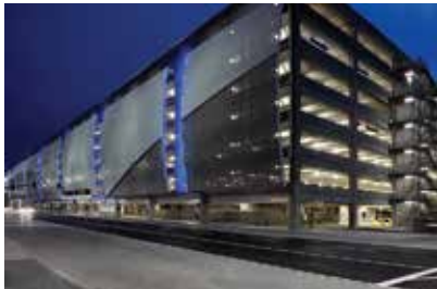
Dramatic photography was used as an aesthetic treatment for the San Jose International Airport CONCRAC structure, which features a total precast concrete structure. The technique was still being discussed when the structure was constructed, so designers had embeds placed into the precast concrete that the final decorative pieces could use for installation. Photos: Clark Pacific.
