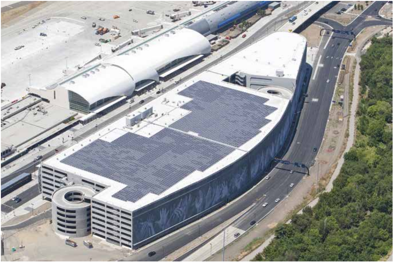
Dramatic photography was used as an aesthetic treatment for the San Jose International Airport CONCRAC structure, which features a total precast concrete structure. The technique was still being discussed when the structure was constructed, so designers had embeds placed into the precast concrete that the final decorative pieces could use for installation. Photos: Clark Pacific.
